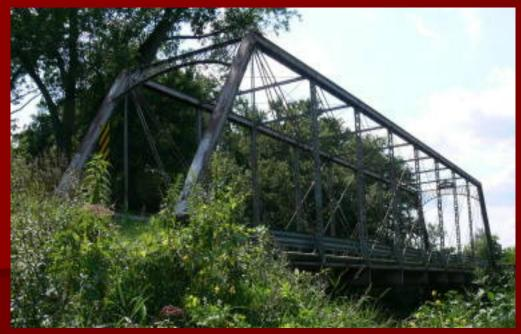
Project scheduled to start summer 2015 and finish in the spring of 2016. Construction process would include disassembling structure and repairing and/or replacing truss members. All truss members will be galvanized and existing stone abutments will be repaired. The current deck may be replaced with a reinforced polymer deck.
